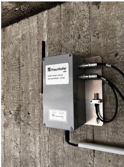
Implementation of "MAUS" on a busy bridge in Munich; © Fraunhofer IZFP
