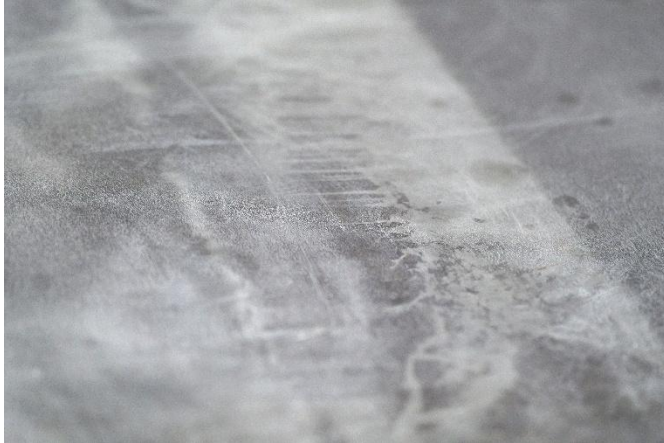
Abb. 3 Used, chemically stripped roof with galvanized surface: ready for second use.
