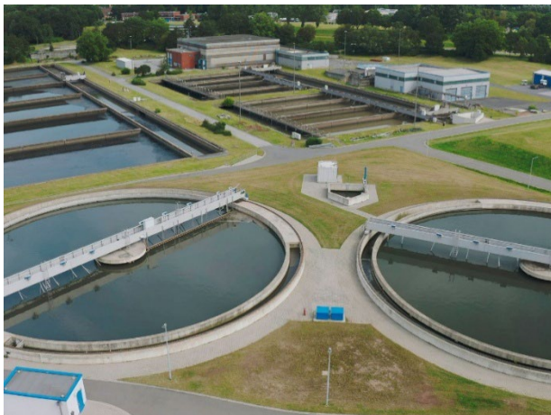
Figure 3 Municipal water treatment plants: Mandatory quaternary treatment will be gradually introduced in the EU by 2045.
