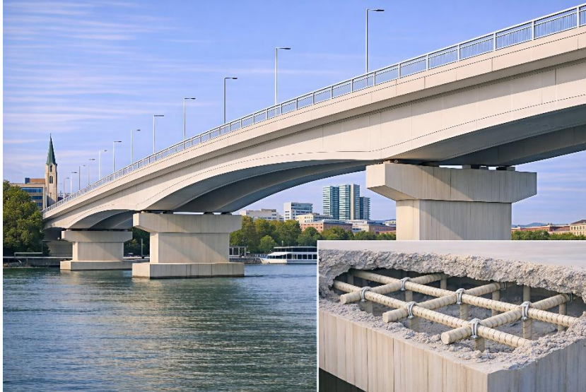
Fig. 3 Alternative to steel reinforcement: pultruded reinforcement bars provide long-term resistance to road salt. © Fraunhofer IWU | AI-generated
