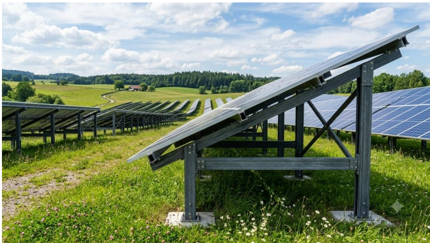
Fig. 2 Does not weather and withstands wind loads: substructures for solar installations made of pultruded profiles. © Fraunhofer IWU | AI-generated
