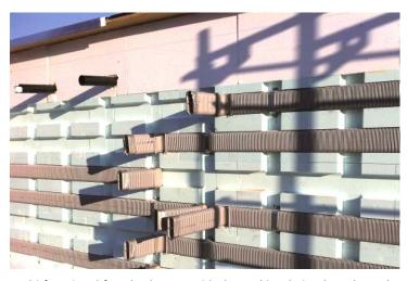
Multi-functional façade element with thermal insulation boards made of polystyrene (EPS) and integrated duct system made of polyethylene (HDPE) ©Fraunhofer ISE
