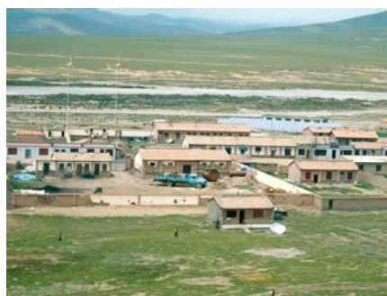
PV-wind hybrid system in a Chinese village. ©Fraunhofer ISE
