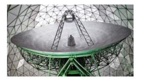
Protected by the largest radome in the world, the space observation radar TIRA has an antenna with a parabolic reflector that is 34 meters in diameter. In spite of its size and a weight of 240 tons, the reflector can be turned 360° in azimuth (horizontal) in just 15 seconds and 90° in elevation (vertical).
