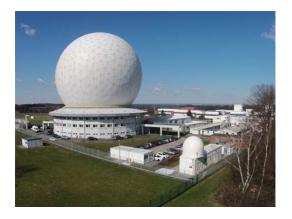
The space observation radar TIRA (left) and the transmit shelter (right) of the space surveillance radar GESTRA, which is currently being developed on behalf of the aerospace management of the German Aerospace Center for the Space Situational Awareness Center of the German Armed Forces. PRESS RELEASE March, 23 2018 || Seite 3 | 4
