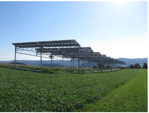
Agrophotovoltaics combines agricultural production and electric energy generation by photovoltaics on the same piece of land. The pilot installation in Heggelbach near Lake Constance, Germany is shown here.
