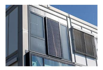
Exterior view of the EE module façade with room-high PV element.
