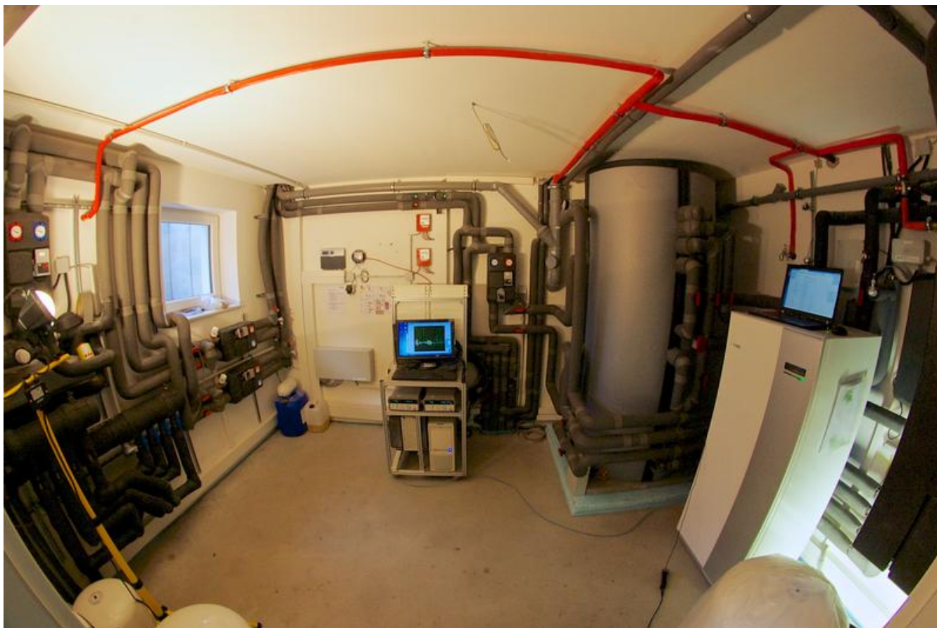
Heating room with measurement equipment (in the center), heat pump and buffer storage. ISFH
