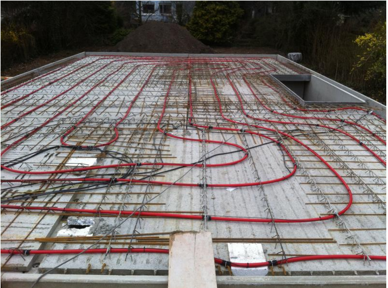
Installation of the thermal activation into the ceiling between cellar and ground floor in the prototype building. ISFH
