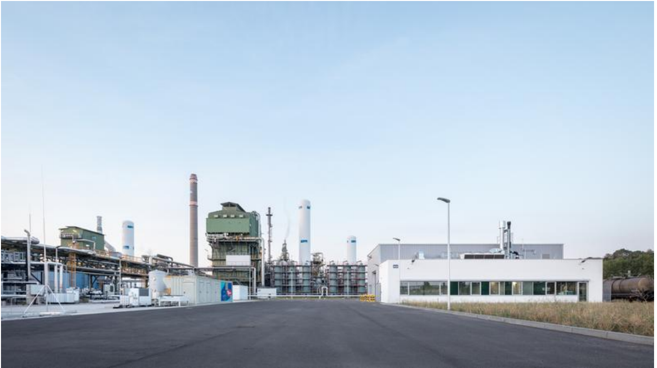
Fraunhofer IWES Hydrogen Lab Leuna © Till Schuster/Linde GmbH - Anlage in Leuna, Hydrogen Lab Fraunhofer IWES
