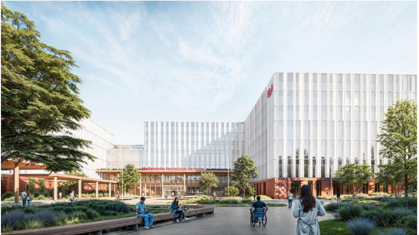
Healing Architecture: The design envisages a light-coloured façade made of recycled aluminium facing the urban Klinikplatz, while the façade takes on a natural character with a warm red colouring on the outside. Copyright: HENN / C.F. Møller
