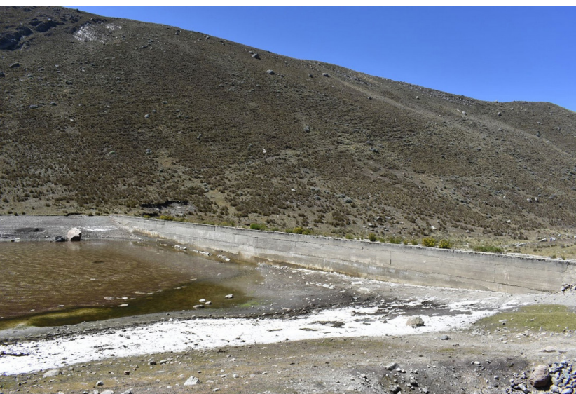
Figure 2. Ricococha Baja: pre-Hispanic dam rebuilt in 2008, failed within six months.
