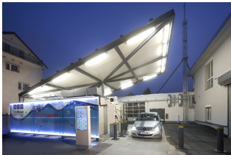
Solare Wasserstoff-Tankstelle am Fraunhofer ISE in Freiburg. ©Fraunhofer ISE
