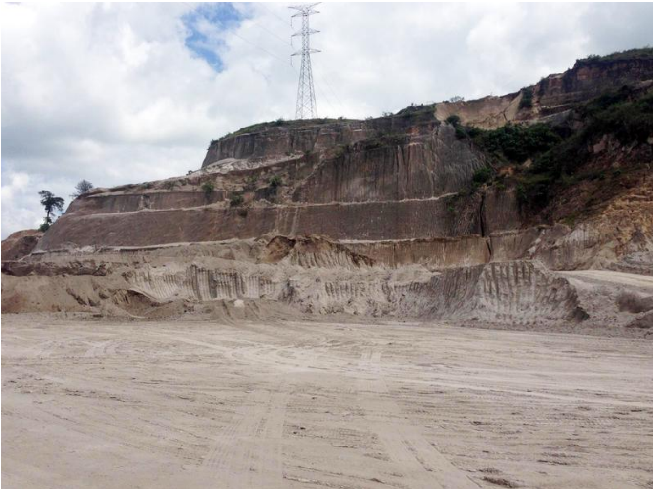
Picture of a pozzolan quarry in Guatemala. There, large quantities of volcanic ash are added to cements in order to reduce CO 2 emissions. Herbert Pöllmann
